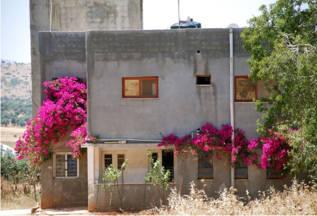
A Typical house in Jalqamous
